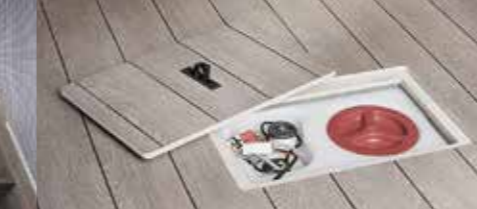
5 Fresh water tank cleaning hatch
